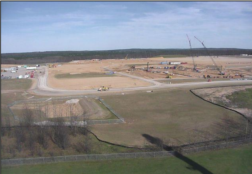
Construction Site of Arauco particleboard plant (May 3, 2017)
